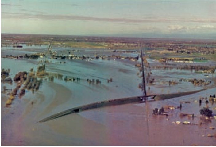
Urbanization on Central Valley floodplains increases risk to lives and property. Photo by Rand Schaal.
