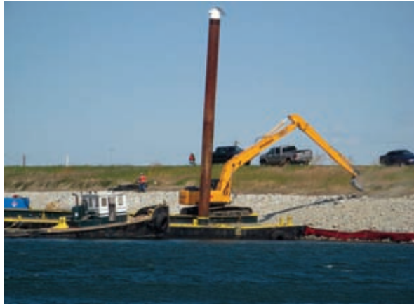
California has relied too heavily on weak levees to protect against flood risk. Photo by California Department of Water Resources.
