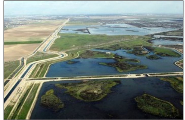
Groundwater recharge basin (Kern County)
