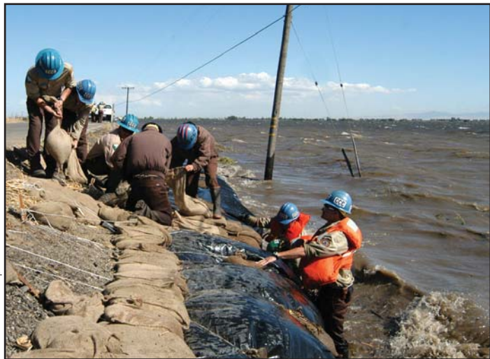
California Conservation Corps repairing the Jones Tract Levee
